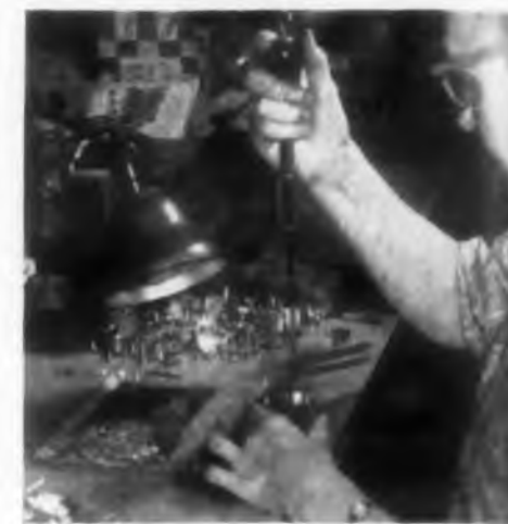
Assembling Hobbs hour meters
