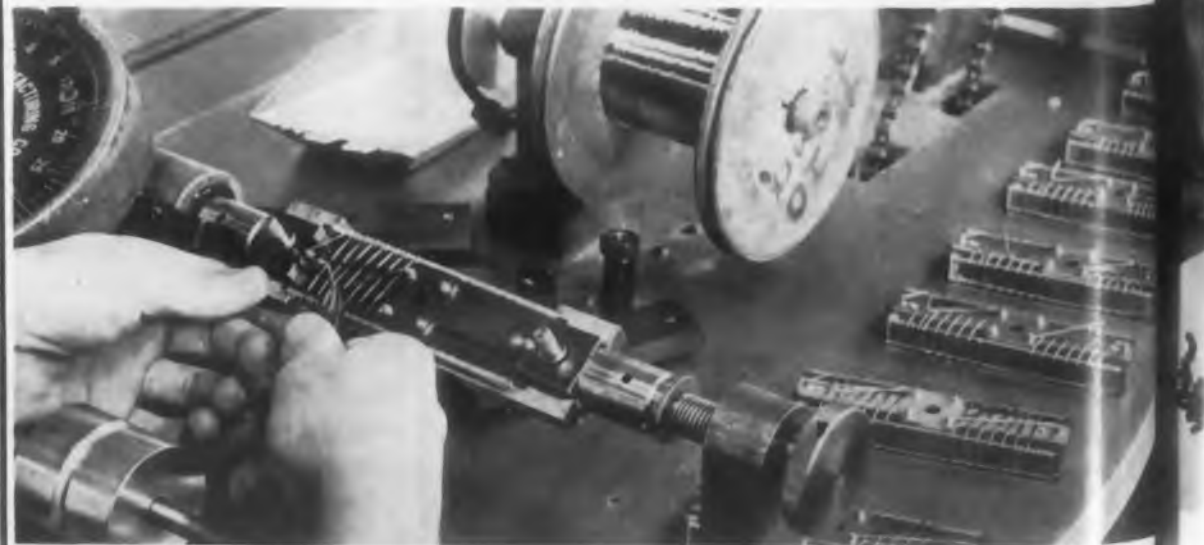
Wire wound ferrite core (shown being wound) replaces "air coil" to give more compact unit with greater sensitivity.
