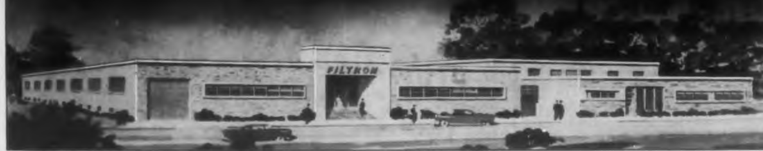
FLUSHING, N. Y., PLANT NO. 1
