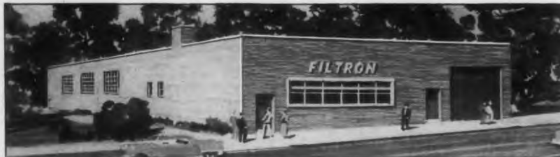
FLUSHING, N. Y., PLANT NO. 3
