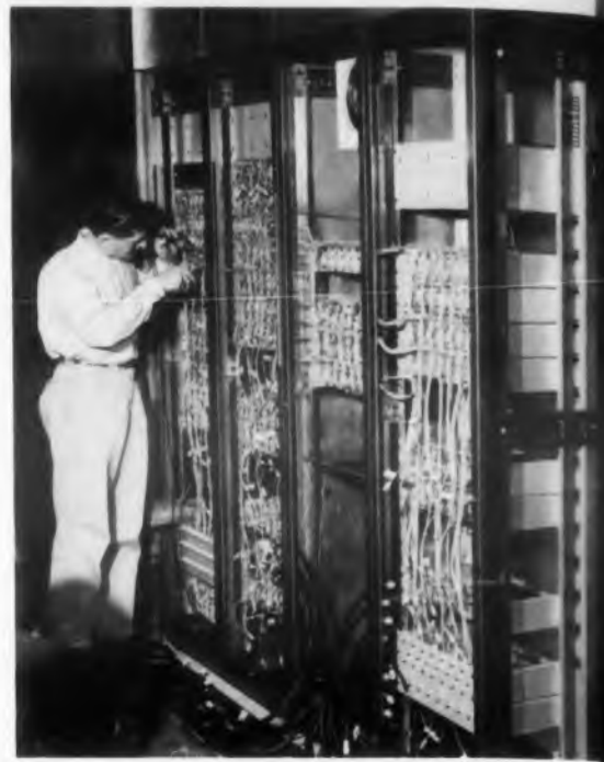
Installing Magnetic Memory For Large Computer
