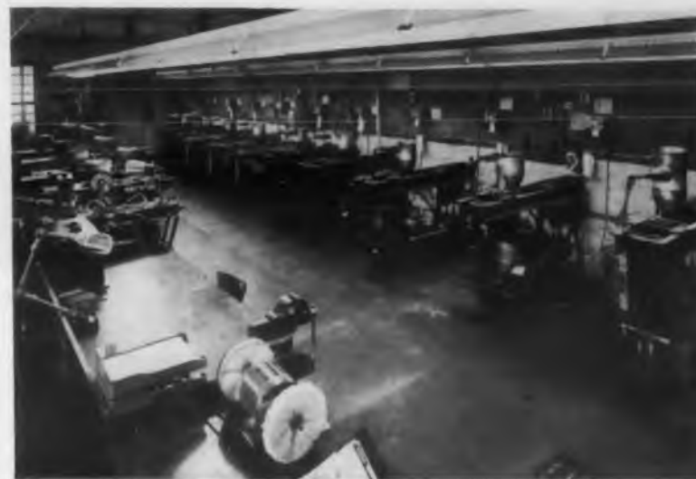
View of a portion of the molding department showing a battery of Grayhill Presses in operation.
