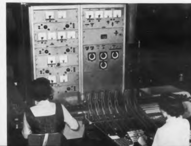
The new Spring City Transistor Plant is unmatched for advanced testing methods. Below is a Philco designed high speed Automatic Test Facility for testing seven parameters of power transistors.
