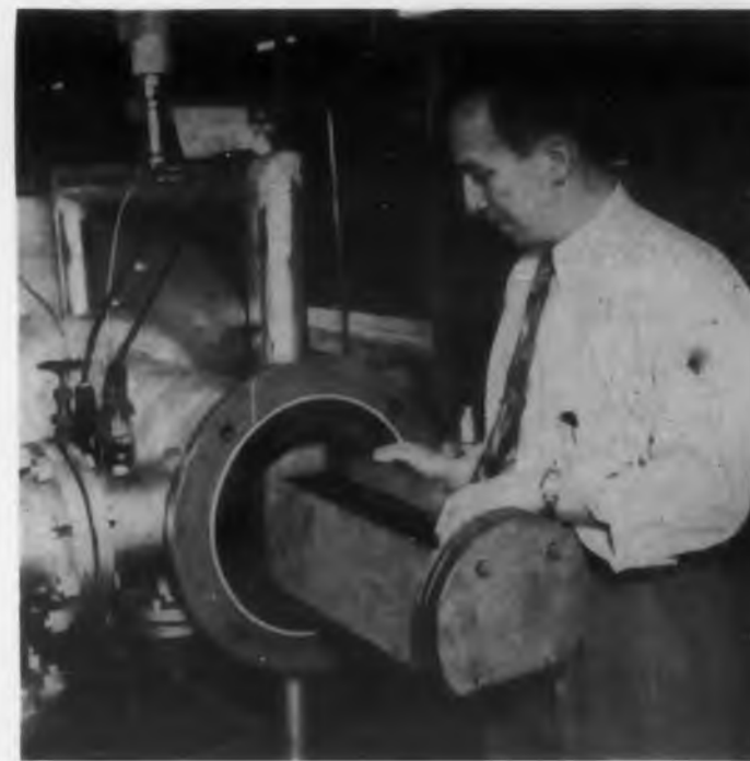
Furnace for heat treating stainless parts
