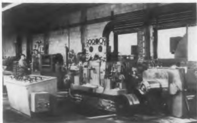
The 16" mill is capable of rolling strip steel up to 13" wide.
