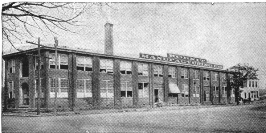
KORNIT FACTORY, NEWARK, N.J. (BELLEVILLE STATION), ENTIRELY CONSUMED BY FIRE, MARCH 1, 1907.
