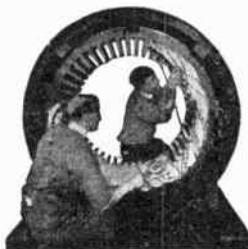
Student winding a Stator
