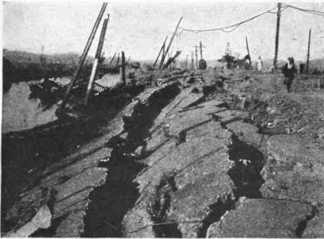
View along a canal through Tokio, as seen after the great earthquake in 1923. Great fissures like these frequently open up in the ground during severe earth tremors.
