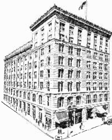
VICTOR BUILDING Our New Building Nearly Opposite U. S. Patent Office Specially Erected by Us for Our Own Use
