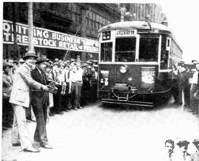
To the left is a close-up of a street car being controlled by radio transmitter held in the hand of Maurice J. Francill, the key being operated by Victor Miller, Mayor of St. Louis. Note receiving apparatus mounted on the front of the car.
