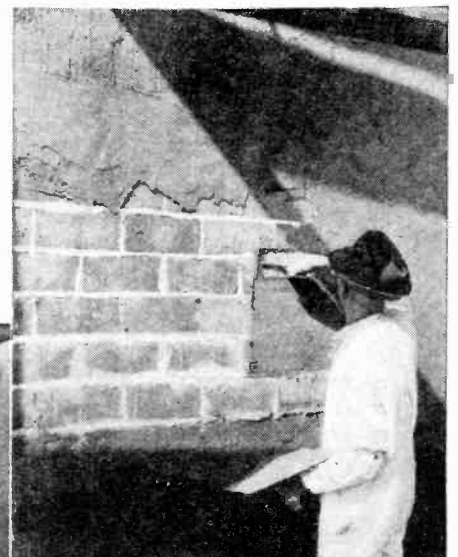
The mixture shown at the lower left contains insufficient cement-sand mortar to fill spaces between pebbles; to the right of it is shown a correct mixture—it will give the maximum yield of concrete. On masonry walls with a coarse texture a scratch coat can be directly applied.
