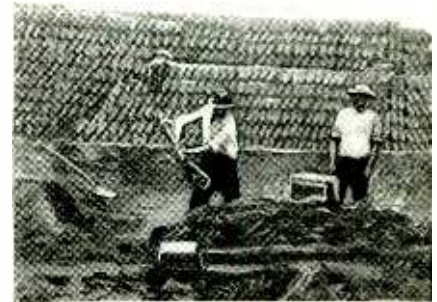
Preparing the adobe blocks.
