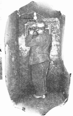
Telephone alcove in a modern mine. Telephone lines connect the various galleries with the surface.
