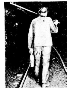
Photos like this, showing how bar may touch trolley wire and cause death, are used to warn miners.
