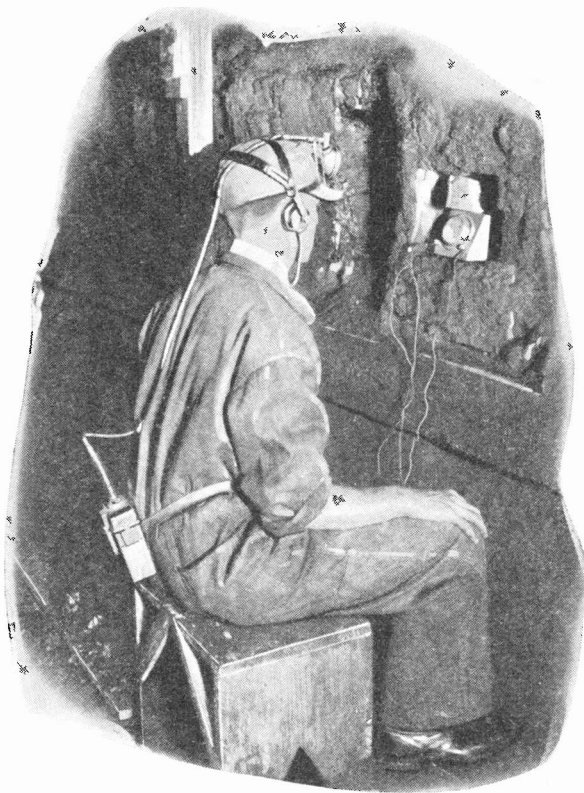
Listening, by means of sensitive instrument, to sounds in another part of mine.
