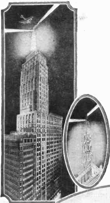
How the Roanoke Tower in Chicago will appear when the aerial beacon is complete. One searchlight always points to the city's landing field.
