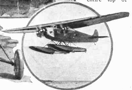
Commander Byrd's plane, which he will take with him on his Antarctic expedition, is shown here in its first flying test, after being equipped with the new pontoons adapted to land in the water or on ice.
