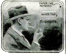
John W. Leon, a student in Columbia University, has invented and perfected a selflighting cigarette. A paper tab treated with an inflammable substance is attached to one end of the cigarette, and when torn off produces a fame. It is claimed that the novel lighter is odorless and tasteless, and will not injure the smoking qualities in any way. In order to light the cigarette, it is only necessary to pull off the paper tab.
