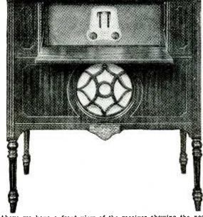
Above we have a front view of the receiver showing the neat panel arrangement and grill work covering the built-in loud speaker. A.C. tubes are used throughout, except on the D.C. set.
