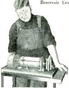
The switch above controls the transmission disks and is governed by a water level float.
