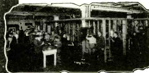
Students Practicing House-wiring In Skeleton Houses.
