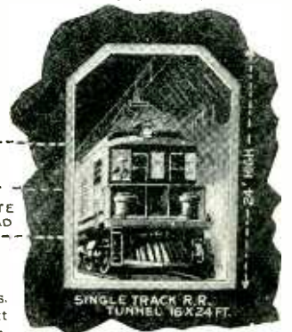
Picture at right shows sectional view through both water and track tunnels. Electric engines will probably be used to haul trains through the Moffatt Tunnel. Cross cuts between two bores will be blocked off after construction.
