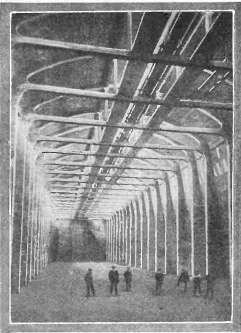
↑ Another triumph of German ingenuity is depicted in the photograph reproduced above. Gigantic halls, constructed entirely of concrete, have been constructed and are in use for the preservation of crude sulphur. All of the supporting beams as well as the cross pieces and other girders are of reinforced concrete. The total length of these halls is in excess of 300 feet, the width is somewhat greater than 60 feet and the height is about 50 feet.
