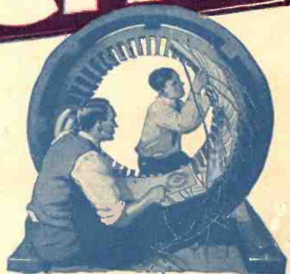
Student Winding Stator in COYNE Shops
