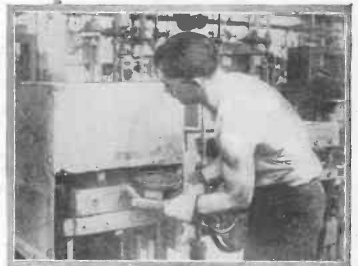
Would you ever think that your dials that control your radio receiving set came from a machine like the one in the above photograph? They do, as this is one of the hot stamping machines that press bakelite or other insulating material into the form of dials. The operator is holding one of the dies in his hand, being protected from the heat by a heavy glove.
