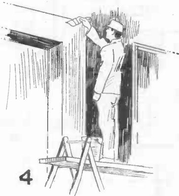
4 Ozonized turpentine makes the paint with which it is mixed dry quickly. It is turpentine which has been exposed to the air and sun light.
