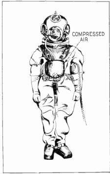
A front view of a modern European diving suit. It has no cumbersome air-hose, the air supply being regenerated by apparatus worn on the back. The life line carries a telephone cable.
