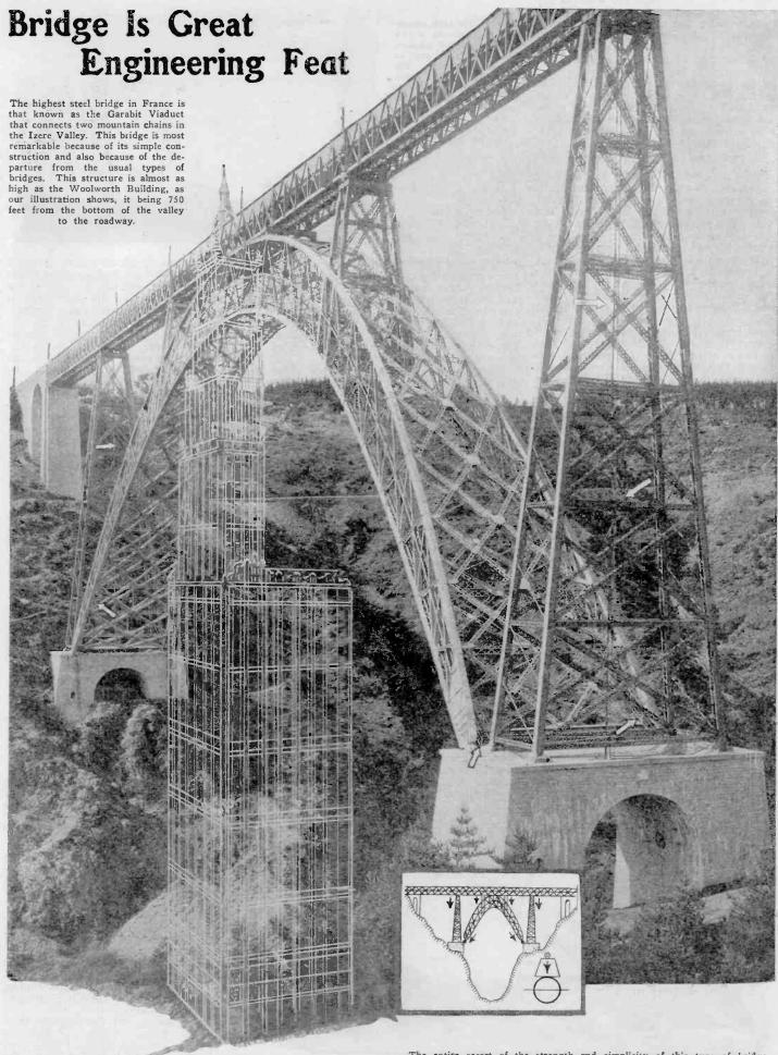
The arrows in the illustration above indicate stairways and ladders that make every part of the framework of this remarkable bridge easily accessible for inspection, painting and repairing. The entire span rests can four concrete abutments.
