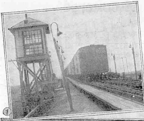
1 Above: View of control tower which also shows a train of freight cars proceeding down the hill toward the switches and car retarder.
