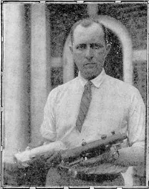
Above: Mr. Swartzel holding one of the rough castings that will eventually be the boiler of one of his locomotives and the wooden form from which this casting was made.
