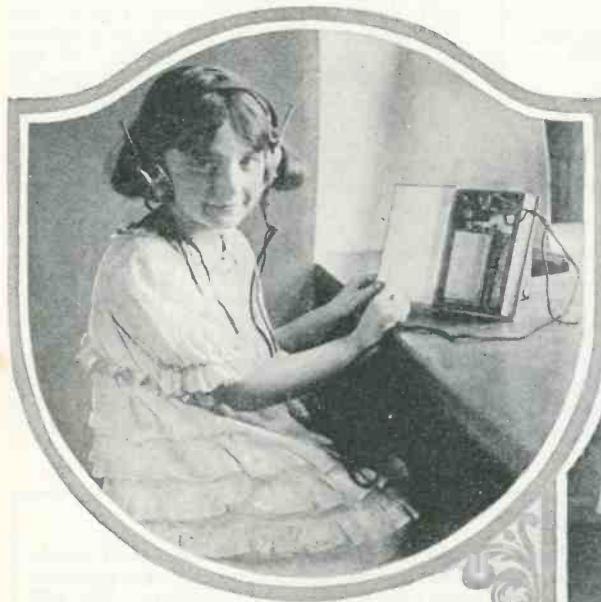
The complete crystal set is clearly depicted in the photograph at the right. The tuning coil is composed of 80 turns of No. 22 S.C.C. A slider alongside of it readily tunes it.
