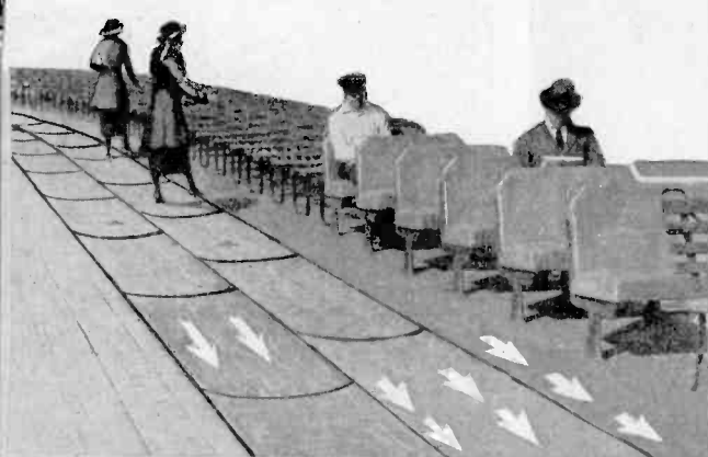
Above is shown a section of the complete arrangement with the three moving platforms. The slots marking the connection point between the sections out of which the device is made may be easily seen. Each section is approximately six feet in length. The floors are of wood, the frames of fabricated steel.
