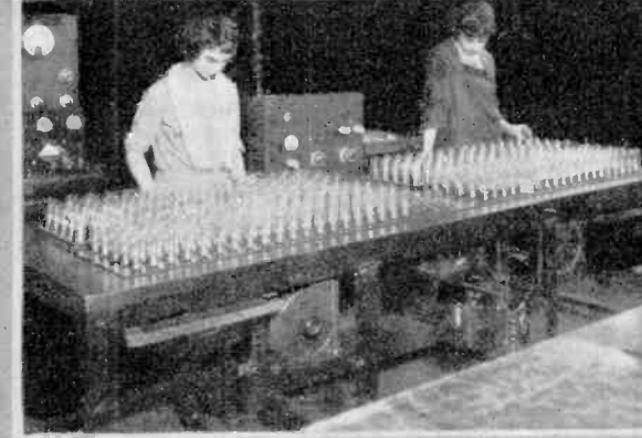
Above is shown the testing table where bulbs are tested for plate and filament consumption. After being burned for an hour on this table, the bulbs are set aside to age and are tested again, whereupon, if they come up to the standard, they are packed for shipment.
