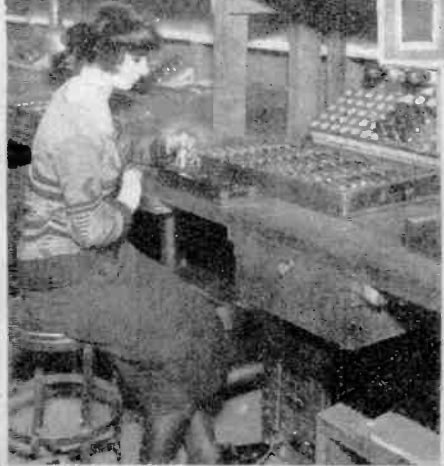
The bases are now sealed on the tubes and the connections made to the prongs. The young lady in the above illustration is testing the connections. At this stage many tubes are rejected because of defects in the filament.
