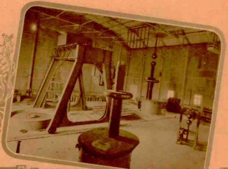
Interior of the high-voltage laboratory of the Westinghouse Electric and Manufacturing Co., at Trafford City, Pa. The huge million-volt transformer can be seen in the right of the photo. This is the only transformer of the kind in the world. A good idea of the size of the apparatus used in the experiments with the so-called artificial lightning can be gained by comparing the size of the man standing by the huge spark gap shown in the extreme right of the picture. A traveling crane has to be used in the building for moving the various pieces of apparatus from one part of the laboratory to another. An even larger gap can be seen just beyond the smaller one. One point of the gap is supported from the ceiling by the huge steel frame-work of the building while the other is mounted on a great insulating pillar. The noise of the sparks released by the high potential currents is deafening.
