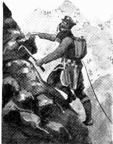
At Left: The New Oxygen Mountain Climbing Apparatus In Use. This New Oxygen Breathing Apparatus Will Make Successes of Mountain Climbing Expeditions Where Heretofore Failures Have Been the Rule. Below: The Apparatus For Inhaling Oxygen From a Single Cylinder.
