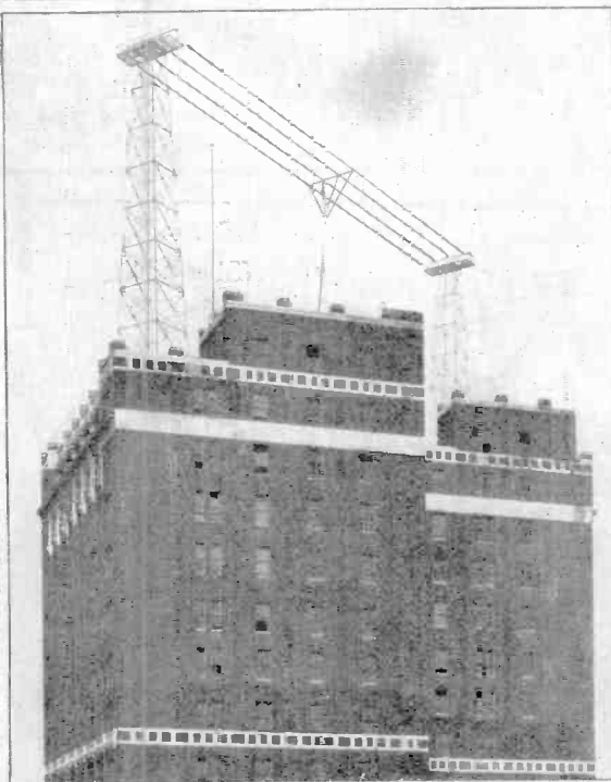
The Photograph At the Left Gives a Comprehensive View of the Aerial and Masts of Station W.E.A.F., of the American Telephone and Telegraph Co., New York City. The Antenna Is Located On the Walker Street Building, and the Studio, a Prospective View of Which Is Shown Above, Is Located At 19 1/2 Broadway.
