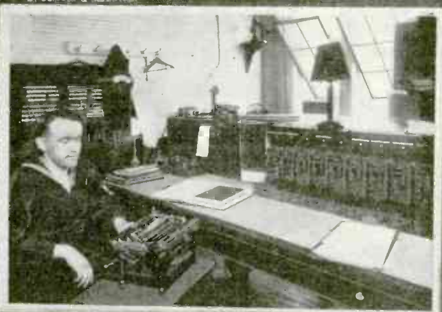
In the left background of the above photo may be seen the switchboard connecting with various points along the Atlantic coast. On the right hand side of the picture are the relays and keys used in connection with these lines.
