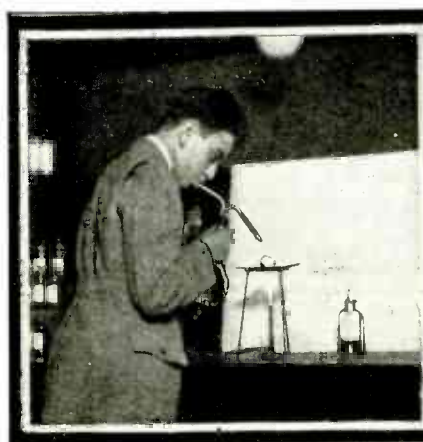
Slaking a sample of quicklime.
