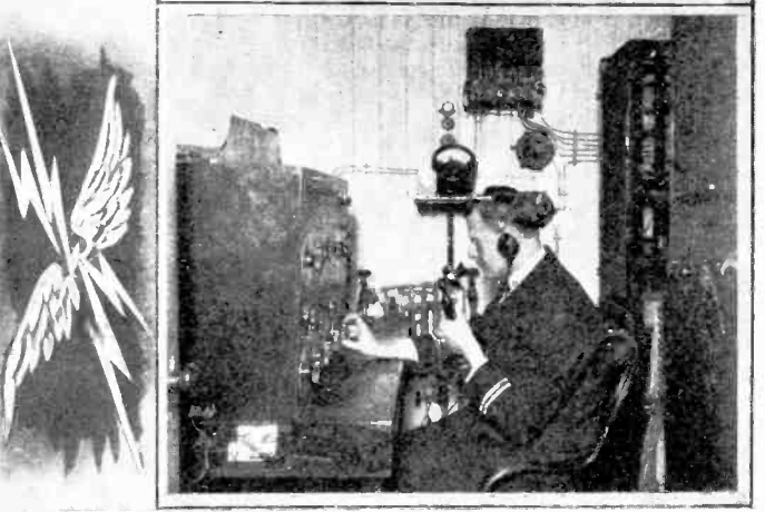
Radiophoning from Ship to Shore and from Shore to Ship Has Become an Accomplished Fact, as was Recently Demonstrated by the Engineers of the A. T. & T. Company. The Two Lower Photos Show the Steamship America from which the Voice was Transmitted to Land and Vice Versa, as well as the Radio Transmitting and Receiving Apparatus on Board the Ship. The Other Two Photos Show the Transmitting Aerial at the Deal Beach, N. J., Station of the A. T. & T. Co., and Also the Interior of the Transmitting Room with the Operator's Desk in the Foreground, the Vacuum Tube Sets in the Background, and the Antenna Connections on the Balcony.
