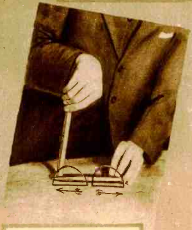
To Magnetize With a Bar Magnet, Stroke the Steel from the Middle With Opposite Ends.
