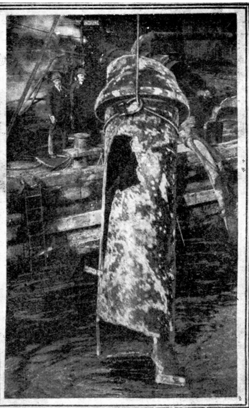
Two Actual Photographs of the Broken 36" Water Pipe Section Which Cut Off the Water Supply of Staten Island Recently. These Photographs Show the Pipe Being Raised from the Water and Also Out of the Water, and the Great Size of the Section Can be Judged from These Pictures. The Water Supply Was Cut Off When the Pipe Cracked, and the Divers Worked in Regular Diving Suits and Cut This Fractured Section of Pipe from the Main Line, 53 Feet Below the Surface of New York Harbor, by Means of the New Combination Gas-Electric Welding and Fusing Device, Shown on the Preceding Page and Also on Our Front Cover. If It Had Not Been for This Electrical Method of Performing the Operation, Much Time Would Have Been Lost and the Cost of Doing the Work Would Have Been Much Greater Also.
