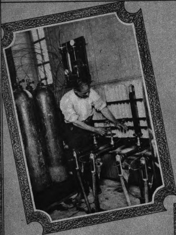
Applying Chlorine Gas at the Kensico Reservoir for Sterilizing the Water Supplied to New York City. The Gas is Received in Liquid Form Compress in Cylinders. The Croton Supply is Treated Similarly and Smaller Plants in the Catskills and Croton Watersheds Treat the Streams Before Entering the Reservoirs.—(Copyright by Keystone.)
