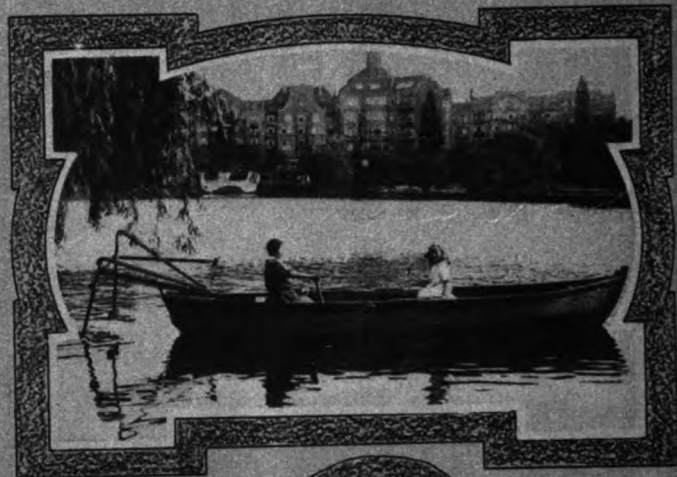
The Paddle Row Boat Worked by Pushing Lever Backward and Forward. No More Losing Your Oars. This Latest Invention Recalling the Canoe Paddle is Very Simple to Work With the Two Arms, Which Also Work Individually. They are Used as Pushers by the Lever in the Seat Not Only Making the Boat Go, But Serving as Good Exercise for the Back and Arms.—© Kadel & Hertel.
