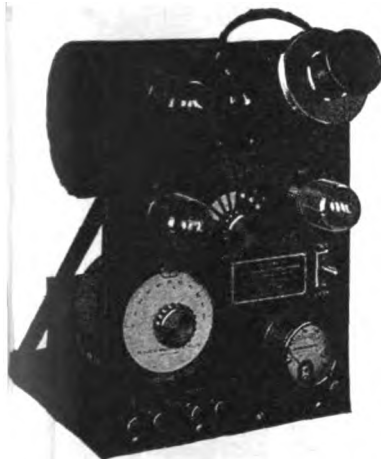
DeForest Portable “Radiophone” Transmitter, Buzzer Type O. T.—5 “Radiophone” Name Copyrighted.
