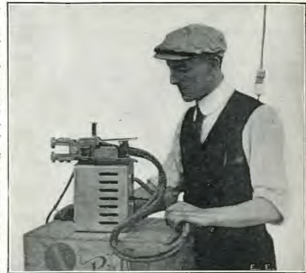
Portable Electric Welder Useful in Sealing Binding Wires on Cases, Barrels, Etc.
