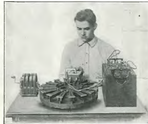
Clever Battery Magnetizer Recharging a Ford Magneto.
