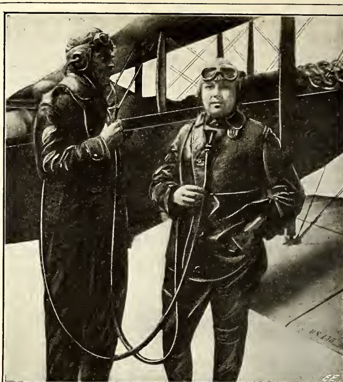
Above:—The Meissner "Airfone" for Talking Between Pilot and Observer. It Amplifies as Well as Localizes the Speech Waves. At Left:—The Ruggles "Orientator". It is Electrically Operated and Gives All the Thrills of Real Flying.
