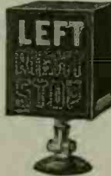
A Logical Design In Electric Auto Signals, Which Can Be Seen from Front or Rear. It is Controlled from the Driver's Seat by Means of a 3-Way Switch.
