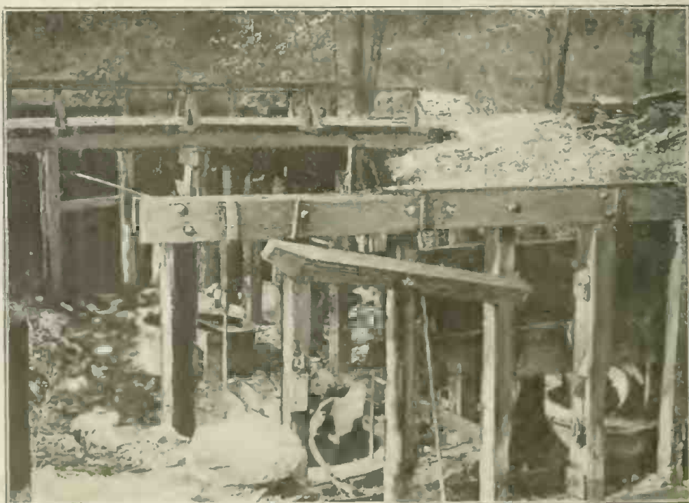
A Remarkable Photograph Showing What Is Thought to Be the Remains of the First Hydro-Electric Plant in the World. It Was Built in 1882, and Started on October 15 of That Year.
