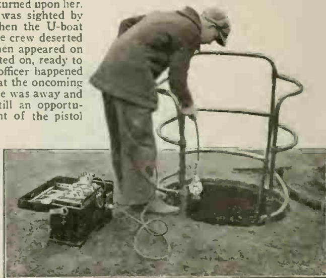
For Lighting Manholes, Cable and Pipe Tunnels, and a Hundred Other Places, This New Storage Battery Lighting Outfit Will Prove Ideal.
