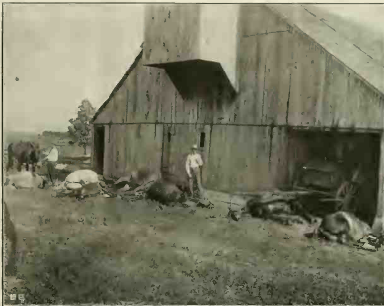
Actual Photograph Taken After a Severe Electric Storm Showing the Lightning's Toll in Valuable Live-Stock. The Barn Was Unrodde, as May Be Surmised, for it is Very Seldom that Fatalities Occur Where Buildings Are Properly Covered with First-Class Lightning Rods, Thoroly Grounded In Damp or Wet Earth.
