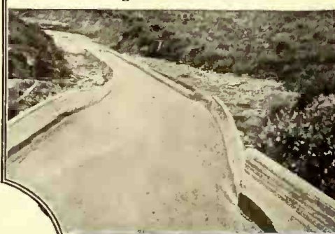
Electric Heaters Prevent This Klondike Gold Mining Stream from Freezing. It Is Six Miles Long and 30 Feet Wide.
