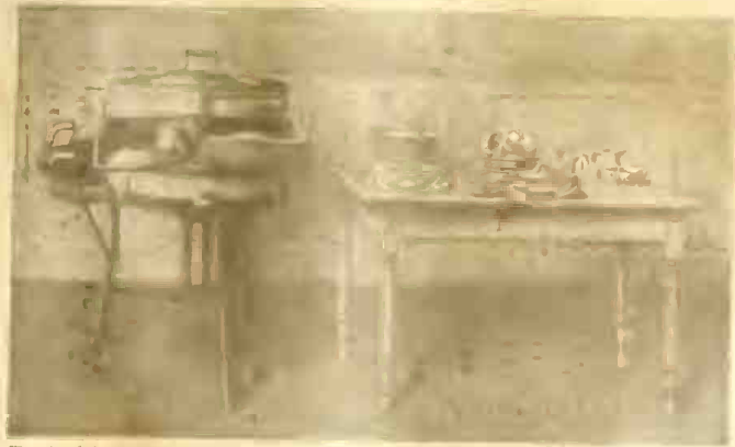
A Typical Installation of a Light Service or Family Size Electric Dishwasher. Suitable for Placing in a Corner Where Economy of Space is a Factor.
