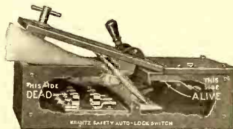
This Switch Automatically Disconnects the Current When the Cabinet is Opened.
