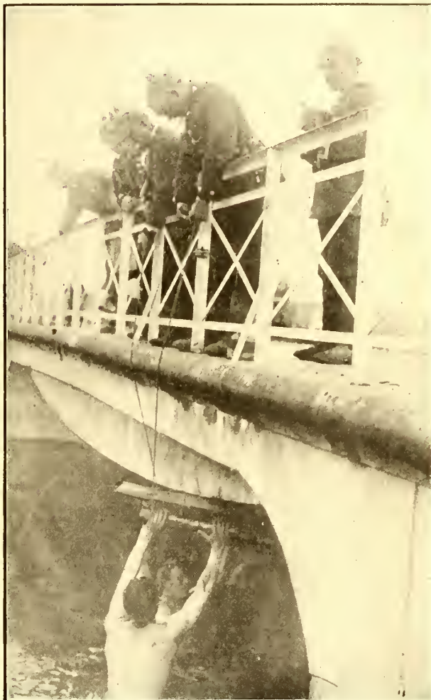
Photos Copyright by Underwood & Underwood. German Military Engineers Engaged in Mining a Bridge. At the Push of an Electric Button This Mighty Structure Will Be Blown to Atoms.
