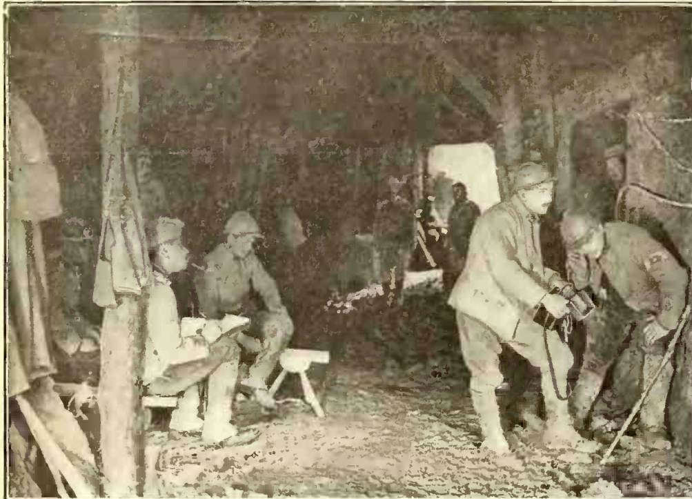
How French Mine Sappers Utilize the Microphone to Hear the Germans Counter-Mining by Sound Conduction Through the Earth.
