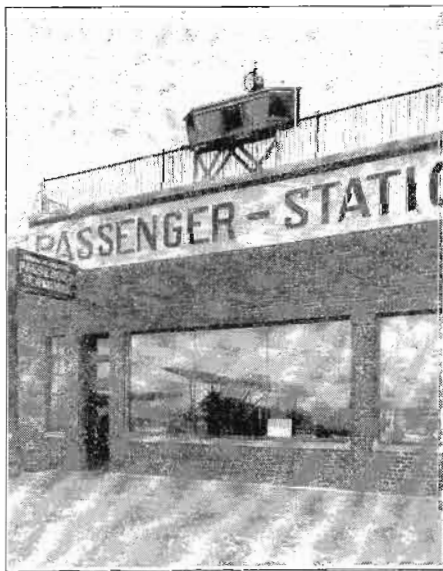
Fig. 5. At the Chicago municipal airport a speech amplifier is used for broadcasting arrival time and messages to the pilot while the planes are on the ground in front of the passenger station. The three Wright DeCoster speakers are shown above the railing in this photograph
