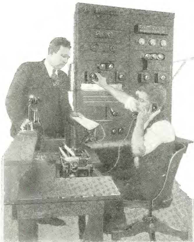
Fig. 11. H. E. Randol, plant manager (standing), and H. Giles, operator, in the station control room. This audio control acts as a link between the studio and the KYW transmitter
