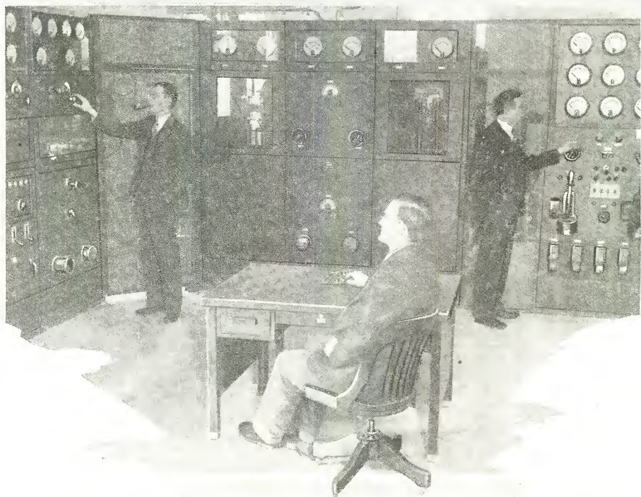
Fig. 14. General view of the new KYW transmitter. H. M. Smith, traveling construction engineer, tuning the 5 kilowatt stage. G. E. Bate at operator's desk, H. E. Randol, plant manager, at right, adjusting filament voltage
