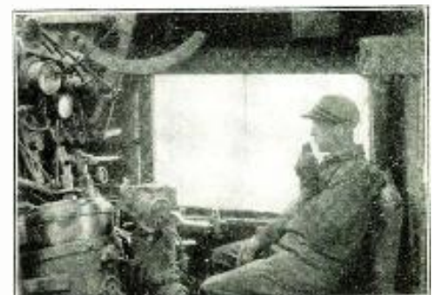
Fig. 8. The engine man is here shown using the microphone of the radio equipment in the cab of a locomotive
