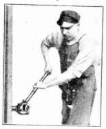
A new rachet type pipe threader, designed for work where a twohandled threader cannot be used.
