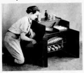
Photo shows the varied uses of stove—baking potatoes and biscuits, frying potatoes, and barbecuing at the same time.
