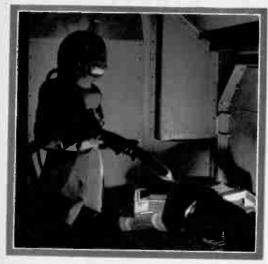
A steel worker pressure blasting castings with a Boron Carbide nozzle with a wearing quality 1,000 times that of an iron nozzle which was formerly used in high pressure work.
