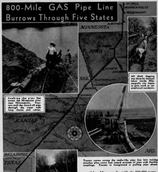
Machines like this cut the 2-foot deep trench for the 800-mile line. Map indicates path taken by pipe through five states.
