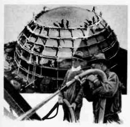
Above—A view of the plantarium dome, erected without costly cement moulds. Inset—A close-up of the mixing and spraying hose used in constructing the huge dome.
