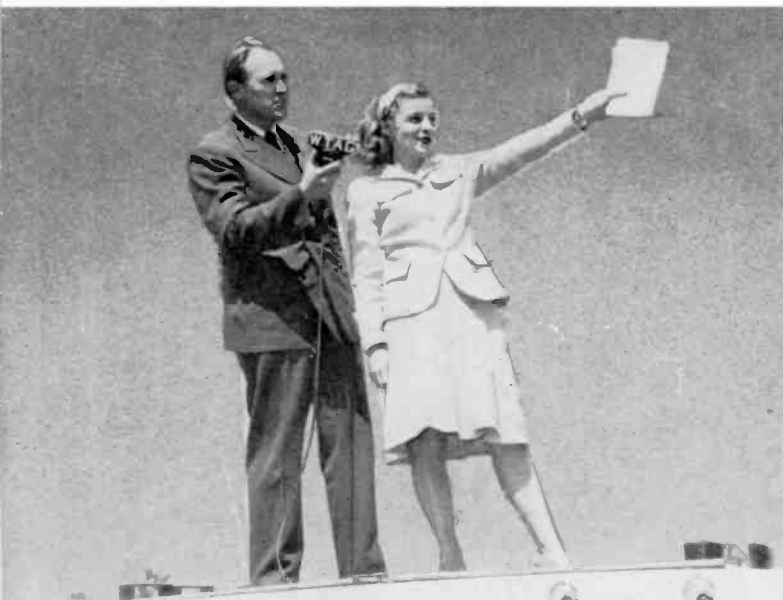
FIRST DYNAMITE BLAST in construction of city's first airport described with "remote" equipment.
