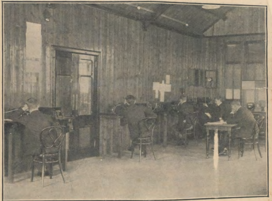
Interior of a Marconi Shore Station.
