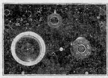
Here we have the front panel view of the One-Tube "Everybody's 100% Low-Loss" Receiver. The large dial at the left is the "Univernier" dial that aids in giving the Cardwell Variable Condenser a fine adjustment. The large knob at the right is the control for the home-made Low-Loss Tuning Unit. The smaller knob at the top center is the Cutler-Hammer Rheostat.
