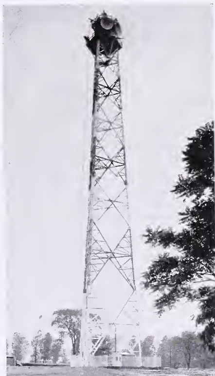
PTM antenna installation at Nutley, N. J., in Federal's multiplex radio relay system.
