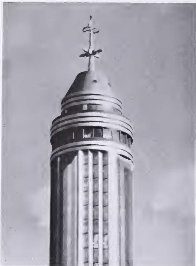
SYMBOL of the Electronic Age: NBC's sight (cross-bars) and sound (ring) transmitting antenna atop New York's Empire State building.
