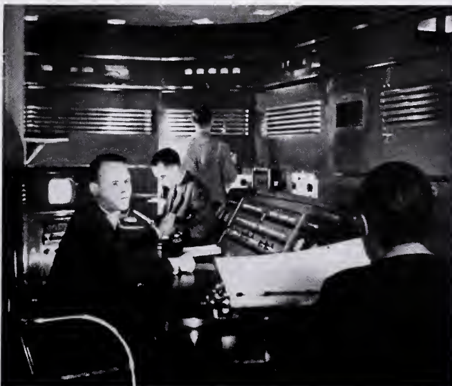
MASTER CONTROL: Technicians watch, hear and regulate the quality of pictures and sound before they go out on the air.
