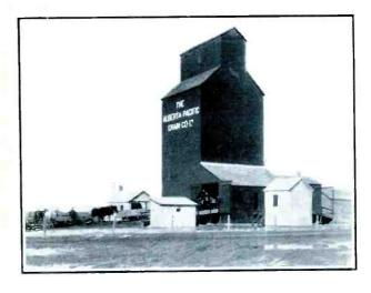
NE of the 550 country grain elevators owned and operated by The Alberta Pacific Grain Company Limited. The average capacity of these elevators is 55,000 bushels of wheat. Each elevator is capable of handling up to 500,000 bushels of grain during the delivery season.
